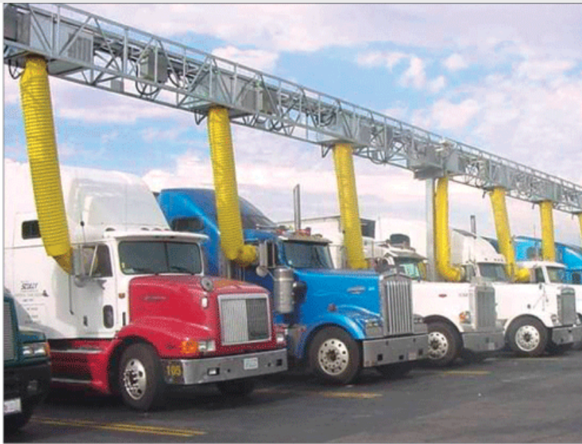
Photo 3. Example of Sharepower equipment
